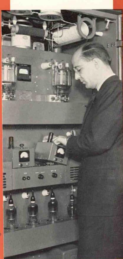
Either oscillator unit can be removed quickly. The selector switch is set to the second unit and transmitter operation continued while the removed oscillator is checked.
